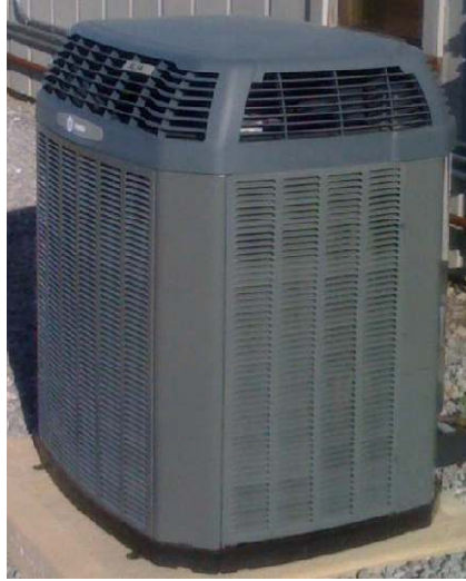
Figure 3.10 Conventional Vapor-Compression System Condensing Unit
