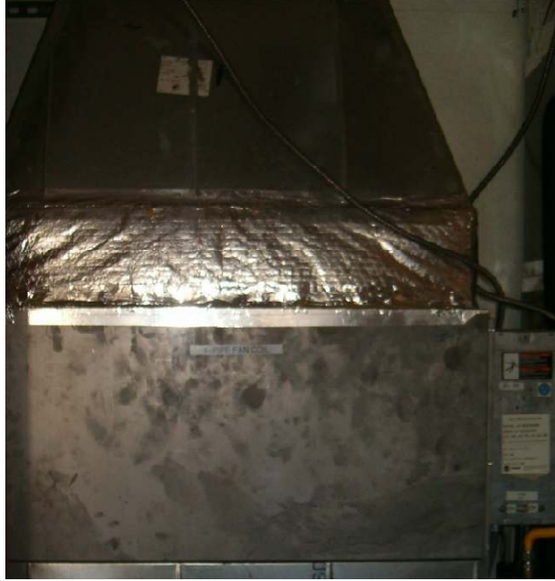
Figure 3.9 Four-Pipe Fan Coil Unit
